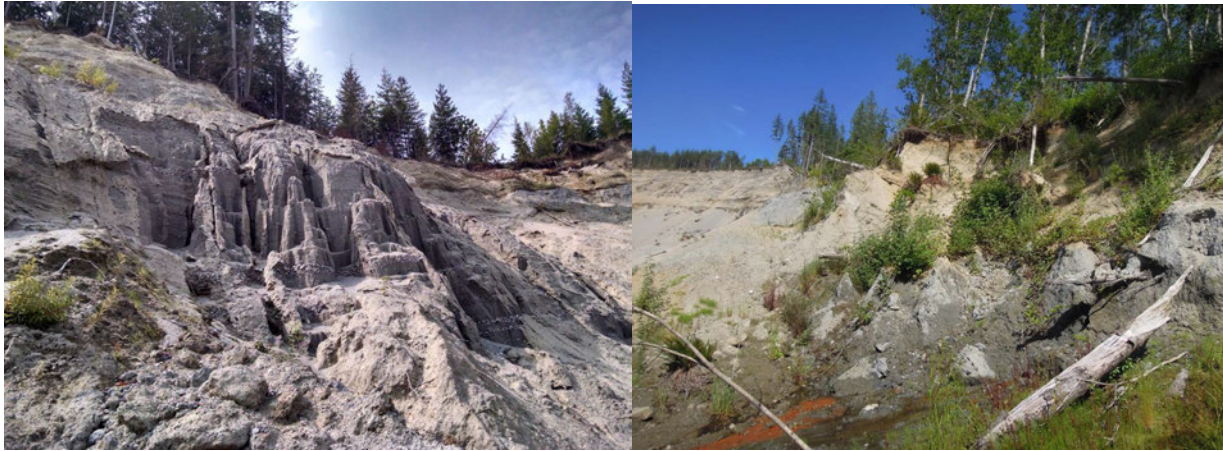
4 5 Figure 27: Western side of the landslide complex shown at the left and eastern side of the landslide complex 6 shown on the right.
