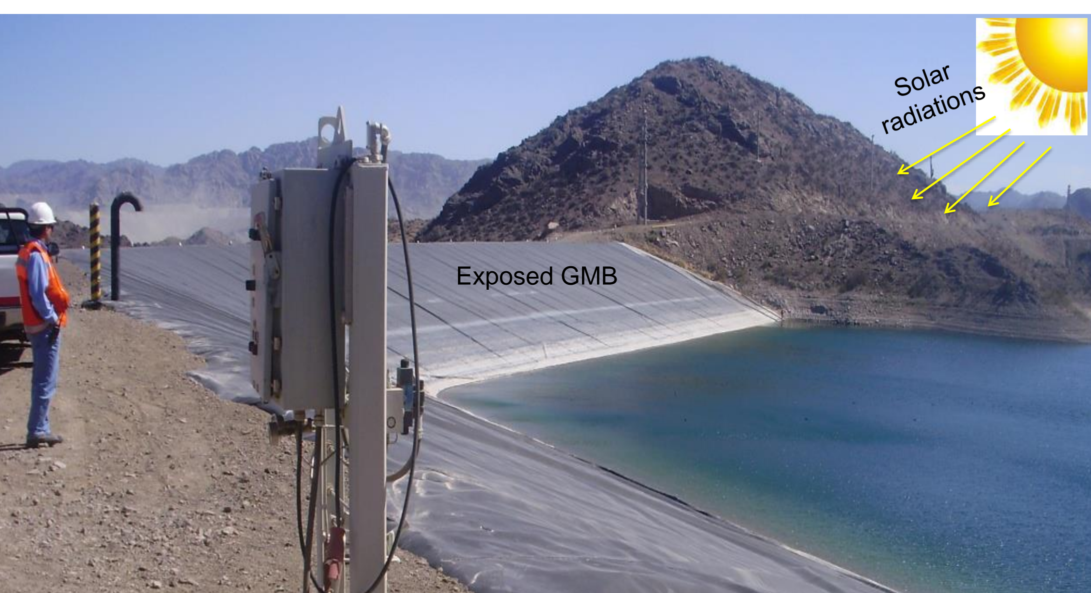
Fig2. Water Dam at Alubrera mine in northwest Argentina [10].
