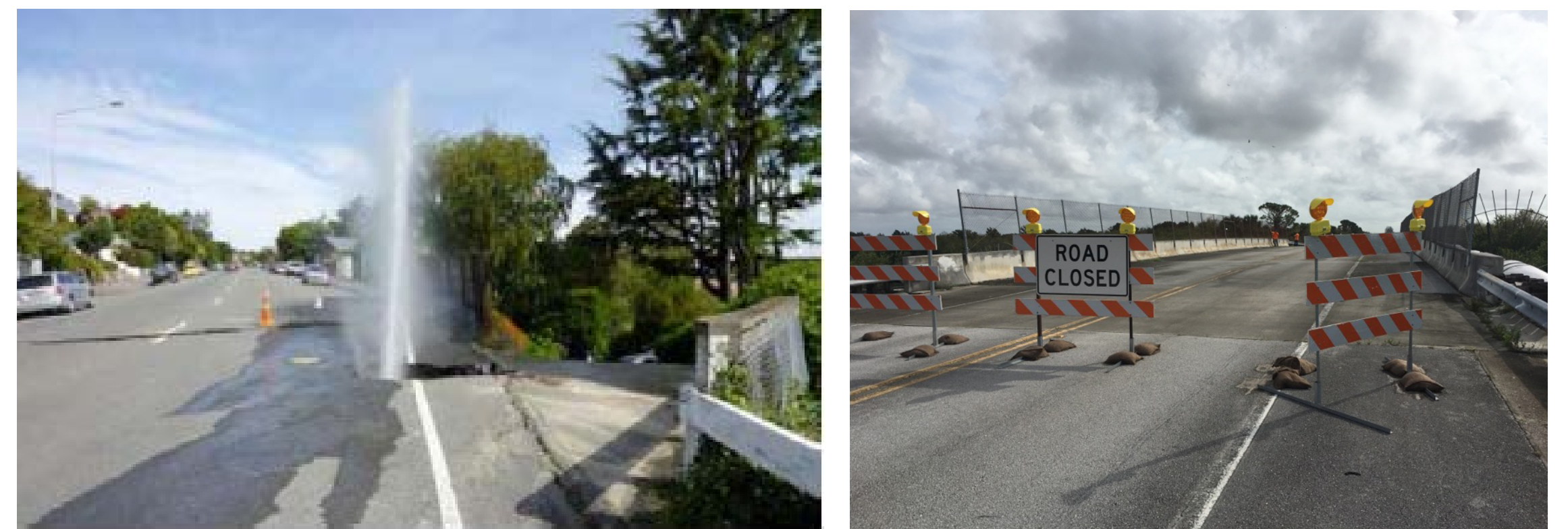
Figure 1. (a) Christchurch, 2011 (Eidinger & Tang, 2014); (b) Syke Creek bridge during Irma (John Campbell/USAC).
