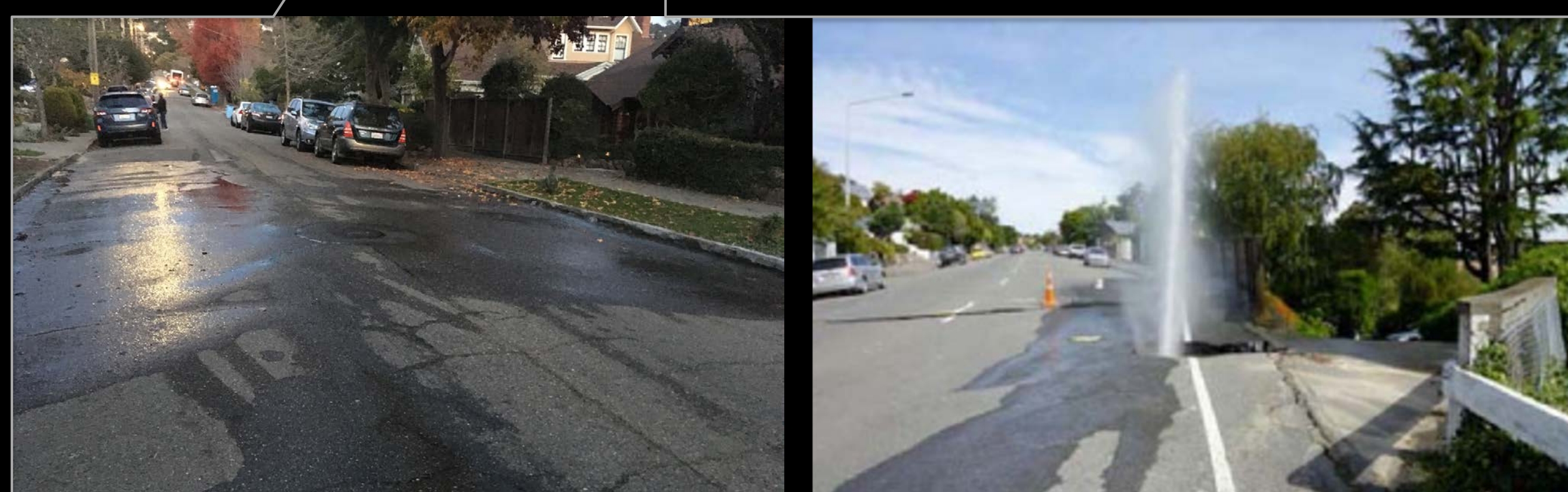
Water pipe breaks. L: Berkeley, 2018. R: Christchurch, 2011 (photo: Eidinger & Tang, 2014).
