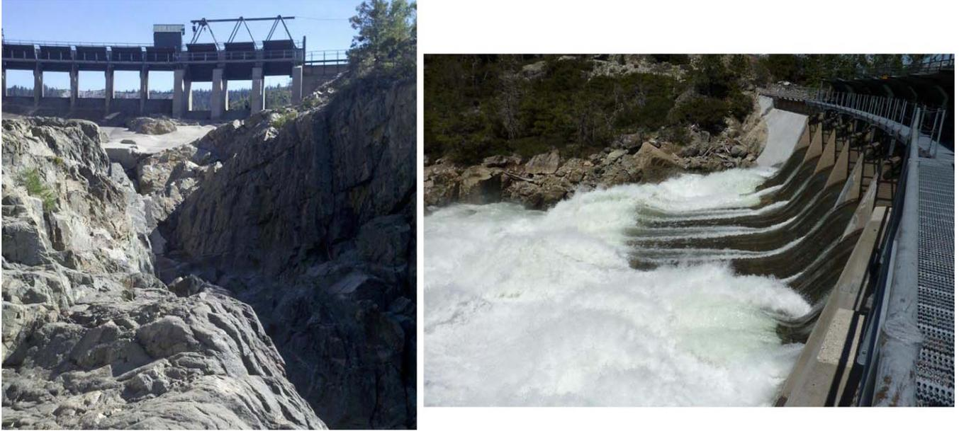
Figure 20: Canyon formed by scour showing spillway gates in background (left). Approximately 2,000 cfs discharge in June 2010 (right).
