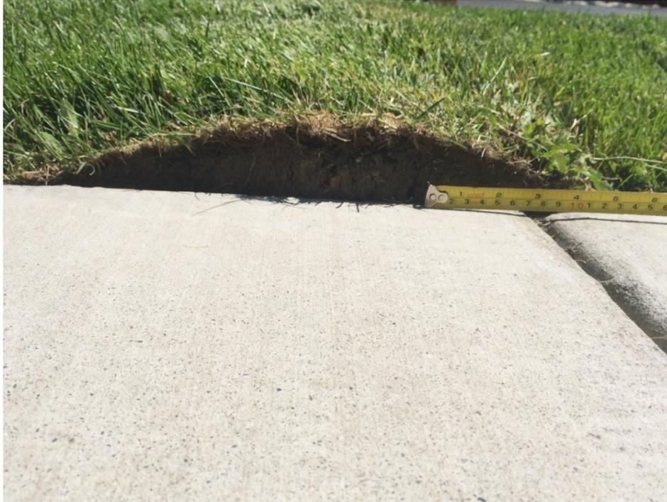
Figure 7: Compression feature in curb strip parallel to fault, across from creek [N 38.3065 W 122.3455; 8/28/2014 13:52]; Bray et al. (2015).
