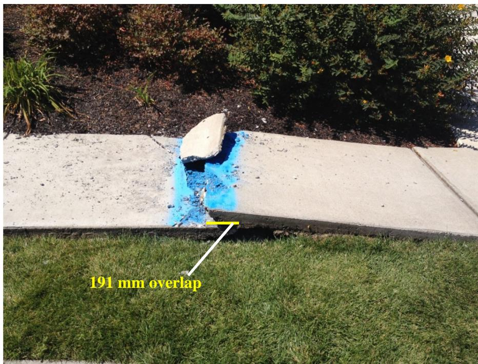
Figure 4: Measuring an overlapped compression zone in sidewalk pavement [N 38.3065 W 122.3454; 8/28/2014 14:00]; Bray et al. (2015).
