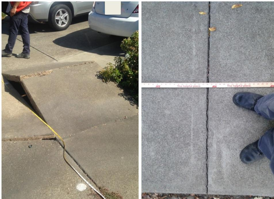
Figure 2: Typical buckled compression zone (left) and extension crack (right) [N 38.3037 W 122.3433; 8/26/2014 15:41 (left); N 38.3055 W 122.3455; 8/26/2014 18:34 (right)]; Bray et al. (2015).
