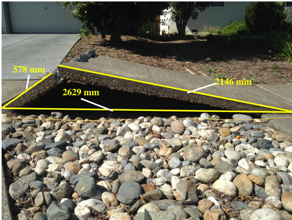
Figure 3: Measuring a typical buckled compression zone in sidewalk pavement [N 38.3039 W 122.3430; 8/26/2014 15:24]; Bray et al. (2015).
